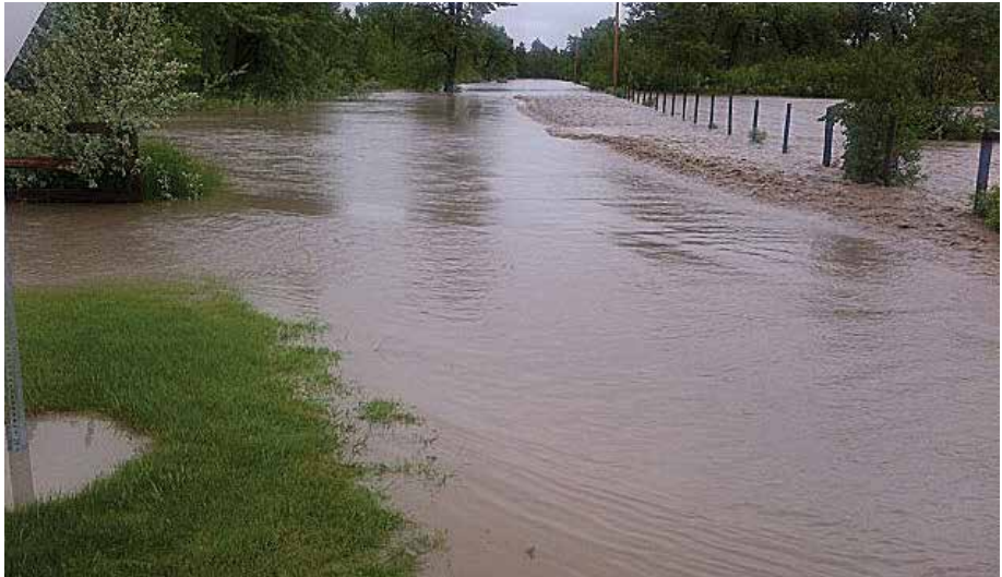
40th Street S flooded
