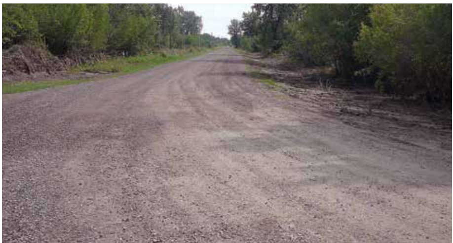
40th Street S after repairs
